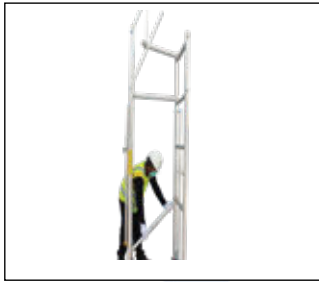
STEP-2 Fit diagonal to connect Podium Frame.
