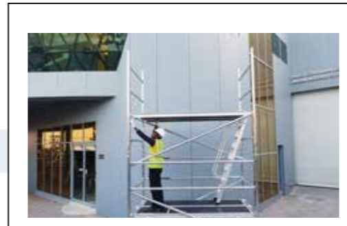
STEP-8 Fit standard and trapdoor platform on 3rd rung from top. Make sure trapdoor door opens to the side of inclined ladder. Engage the wind lock. See Illustration 3.
