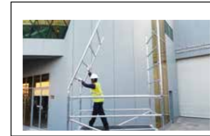
STEP-5 Starting on the guarded platform fit span frame on the lower span frames both the side engage wind lock. See illustration 2.
