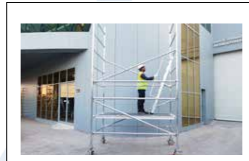
STEP -7 Place inclined ladder with handrail on the platform. Engage wind lock of stairway.
