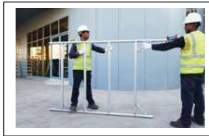
STEP-1 Fit caster in to span frame & ladder frame (or base Frame) and press stop to apply brake. See Illustration 4
