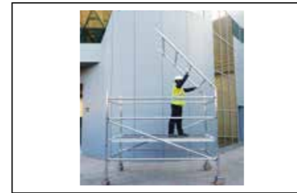
STEP-4 Fit Platform on Lowest rung and fit two horizontal brace on each open sides.
