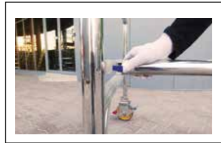
STEP-2 Fit Horizontal brace on the frame lowest rung. Make sure brace hook facing outside from inside.
