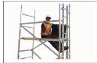
Step 12 Position platform at final height 3rd rung from the top . Ensure windlock system is applied Sitting on the platform fit two horizontal braces on both open sides of platform.
