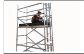
Step 13 Fit the toe board .Slide the side board into the correct slot in the board. Ensuring the object shouldn't fall and trap door opens fully.
