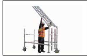
Step 4 Add further frames ensuring the ladder frames are in line.
