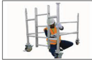
Step 3 Add two horizontal braces, BLUE colour coded, to the vertical member of the frame, as low as possible. All horizontal Brace must fit from inside the tower facing out.
