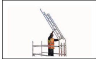
Step 11 Continue to build the tower using the 3T method as step 4,5,6, 7,10. Till the desired height is achieved.
