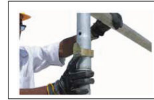
Step 5 Engage Snap pins to the frames (As Illustration 2)
