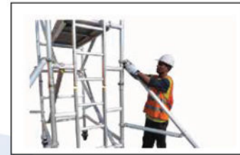
Step 9 Add four stabilizer to the structure at the earliest opportunity. Position the stabilizer so that the footpads are approximately equidistant from the other 45° for maximum stability, ensure lower arm as horizontal as possible.
