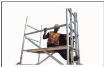
Step 10 Sitting through the trapdoor add two horizontal braces on 5 th & 6 th rung ,two each on both end of the frame.
