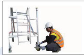
Step 8 Check with the spirit level on both length and width, side of the tower, adjust the wheel if it is required to level the tower, with an inclination of 1%.
